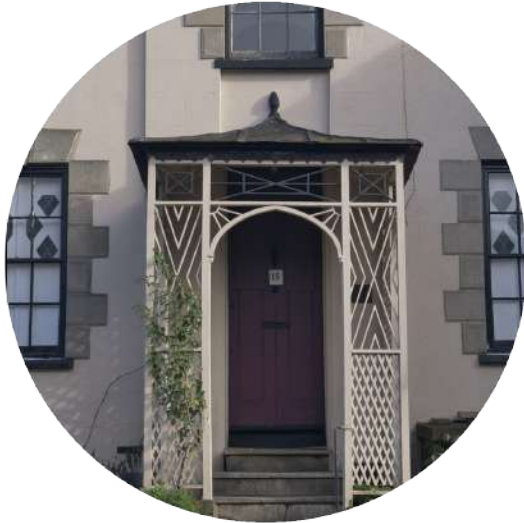
Original six over six sash windows
