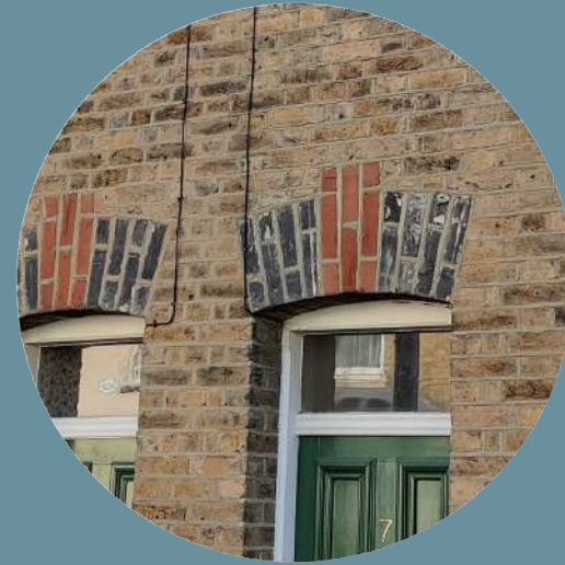
Arched lintel with contrasting brick keystone
