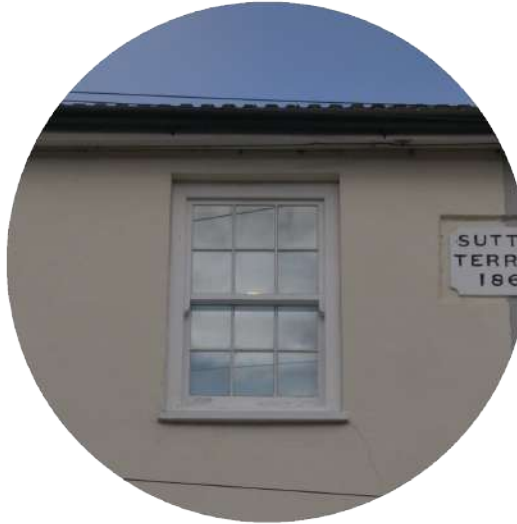
Modern six over six sash window
