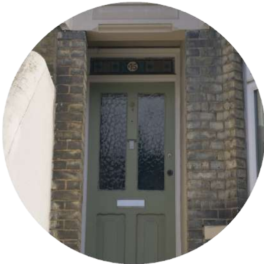
Victorian four-panel door with stained glass transom light
